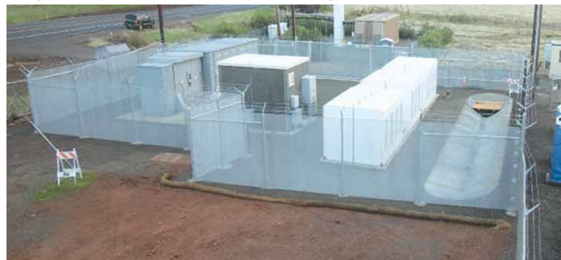
This battery storage system in Brown's Valley is PG&E's first lithium-ion energy storage facility and features Tesla Powerpack technology.
