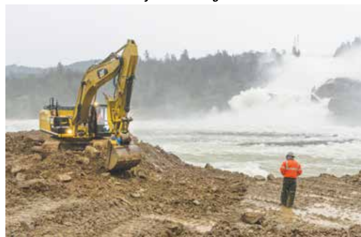
Cleaning out debris below spillway.
