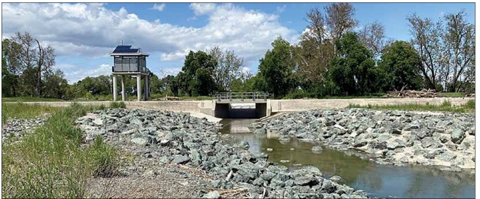
This is the second year the Fremont Weir Adult Fish Passage has operated. Due to drought conditions, the facility was last operated in the winter of 2019. Photo courtesy of DWR.
