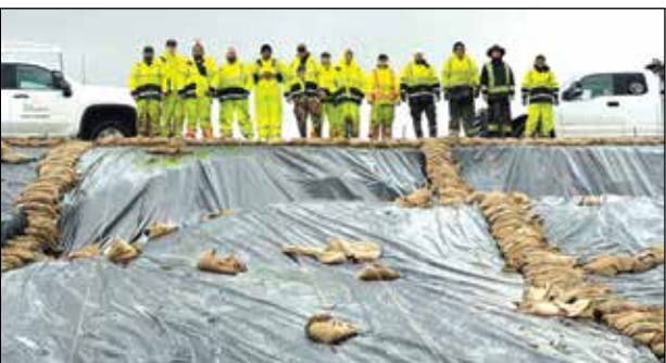
City of West Sacramento public workers use tarps to limit moisture which can saturate the clay in the levee system and cause slumps. Photo courtesy of City of West Sacramento Public Works
