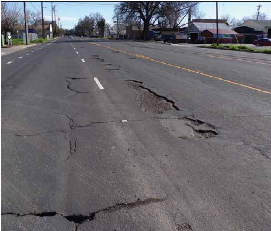
Potholes on Sacramento Avenue show how parts of the road are sinking. Photo courtesy of City of West Sacramento
