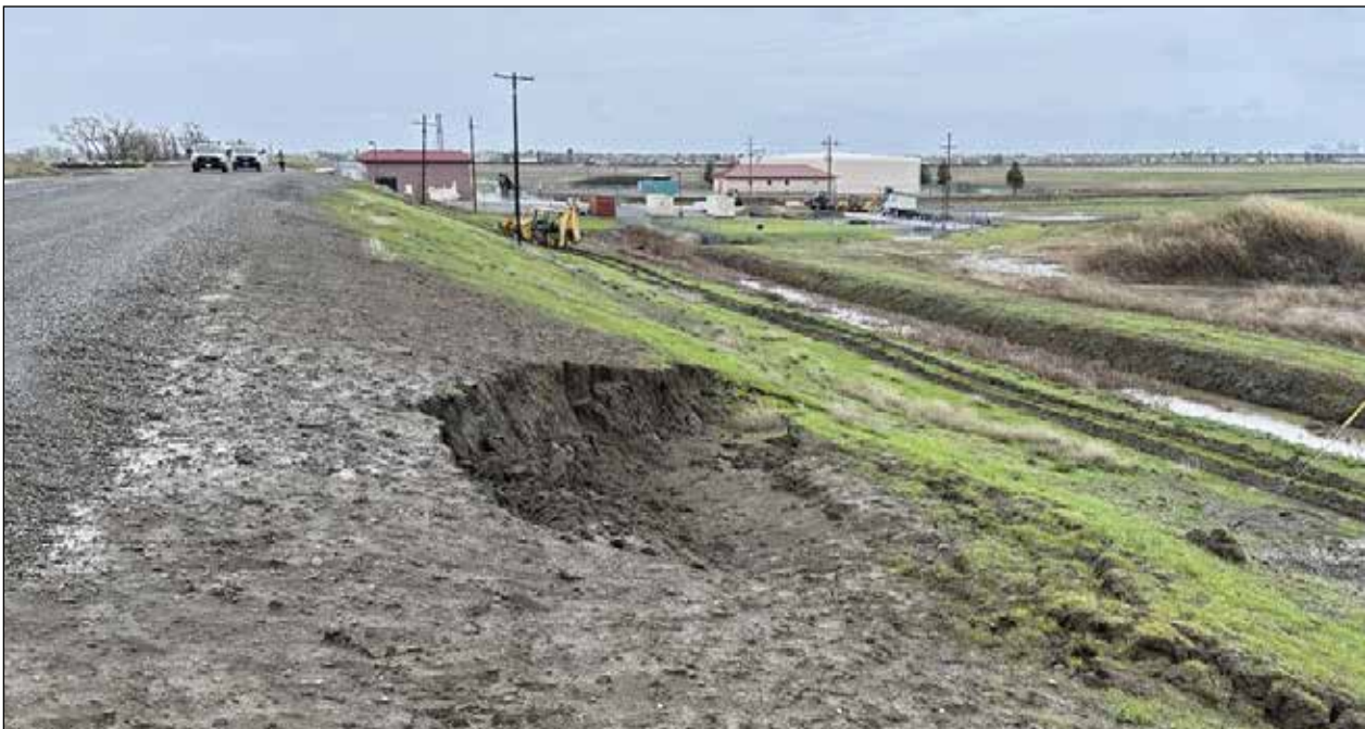
West Sacramento levees have experienced some natural erosion as seen in this slump near the Deep Water Ship Channel. Photo courtesy of City of West Sacramento Public Works
