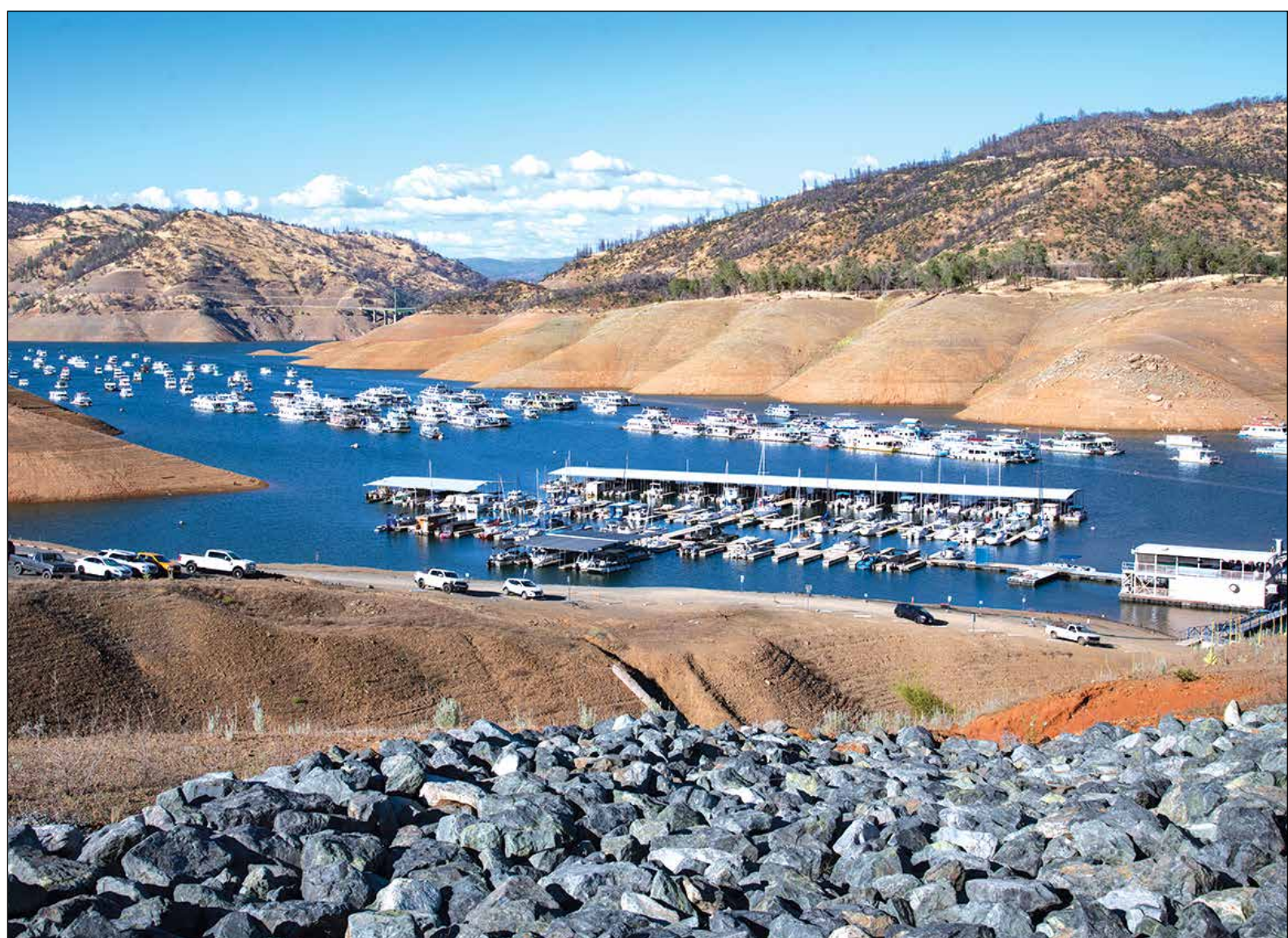
Bidwell Canyon Marina showing Lake Oroville with a reservoir storage of 1,663,134 acre-feet (AF), 47% of the total capacity. Lake Oroville is located in Butte County, California. Photo taken July 6, 2022, by Florence Low/California Department of Water Resources
