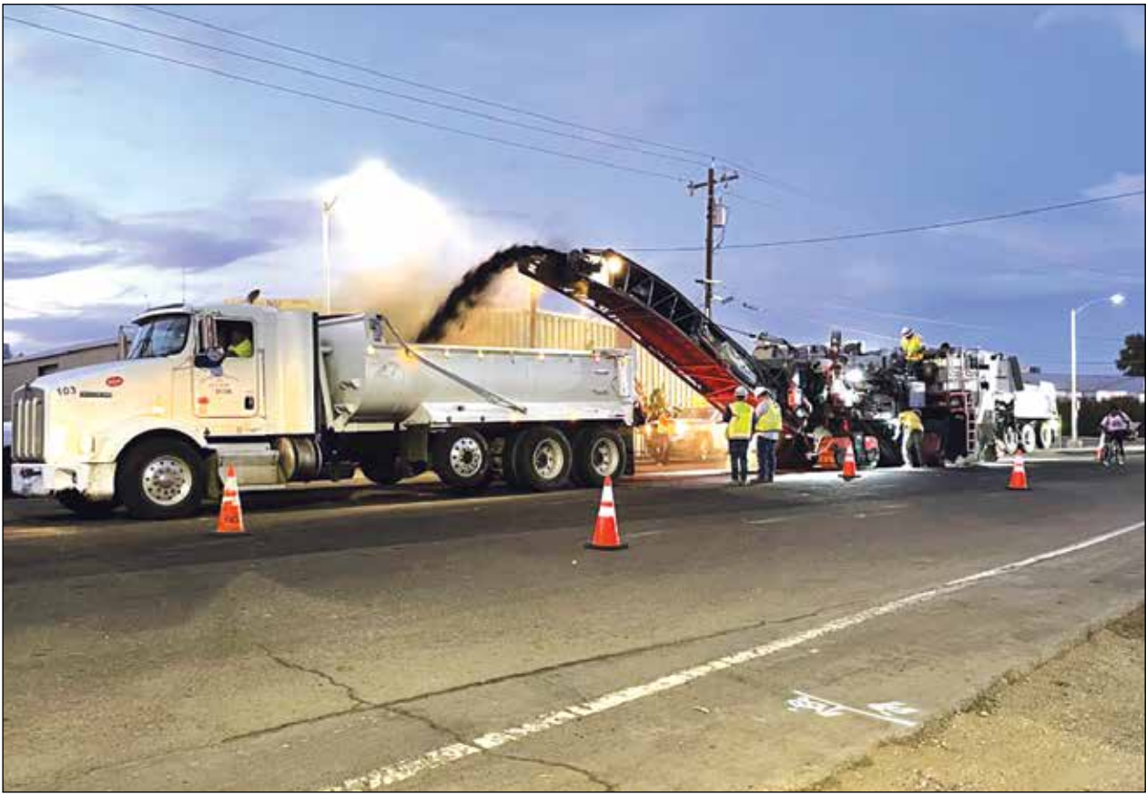
Image of West Capitol Ave undergoing pavement milling thanks to local, regional and SB1 funding. Photo: City of West Sacramento
