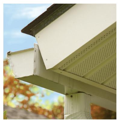
weight. Replacement of separated gutters may or may not be necessary depending on how big the problem is and the condition of the existing gutters. If replacement is not necessary, separated gutters may be remedied by securing the joints, another relatively simple and inexpensive fix.
