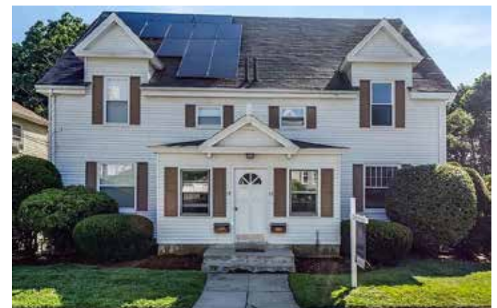
The 6-bed, 4-bath, 3,004 sf house at 13-15 Grant Street in Milford recently sold for $702,000. Photo credit www.zillow.com
