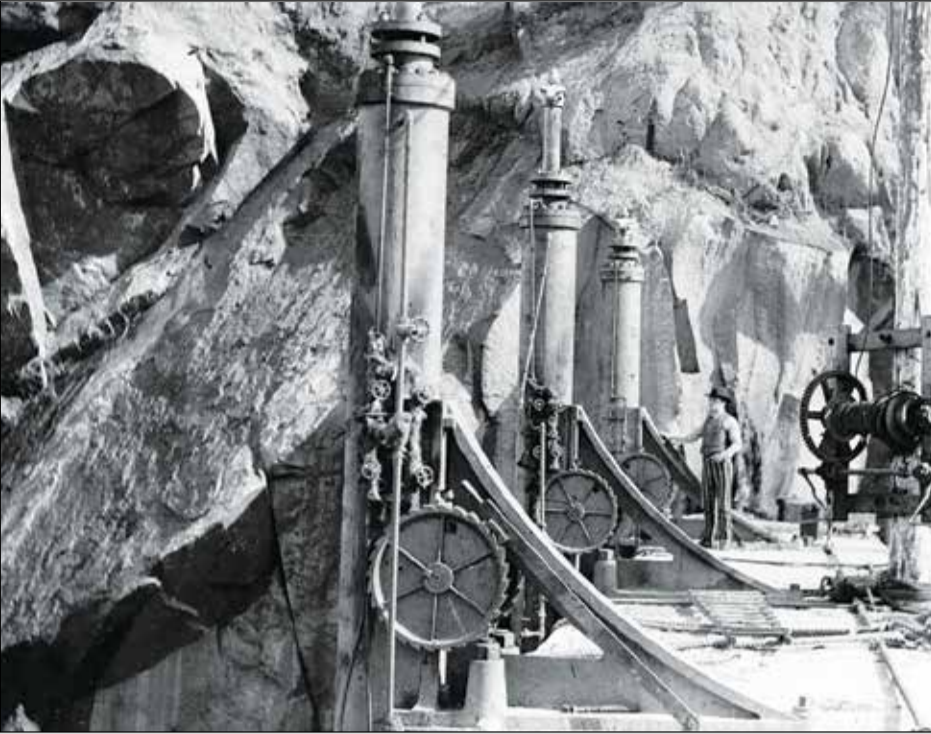
The old Folsom Dam's gates are a great depiction of machinery to human scale. Photo courtesy of California State Library's Folsom Prison collection.
