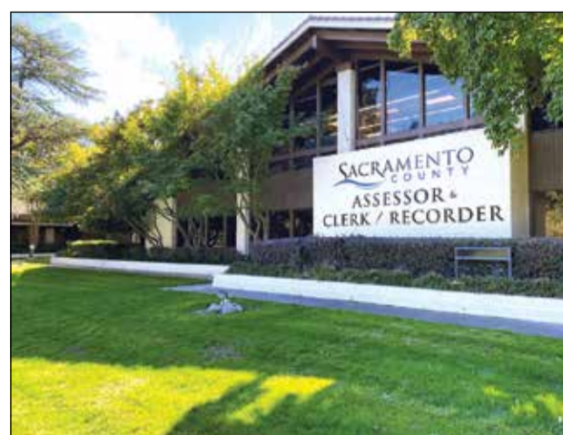
The new central office is located at 3636 American River Drive in the unincorporated part of the County near Watt Ave and Hwy 50. Photo courtesy of Sacramento County
