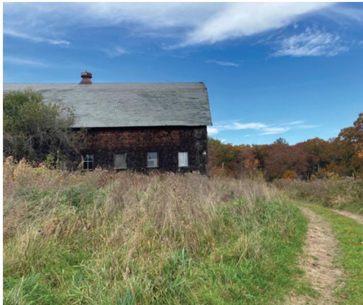
Although the house at the parcel known as Schmidt's Farm will be demolished, town officials hope to find a way to preserve this barn for future use.
