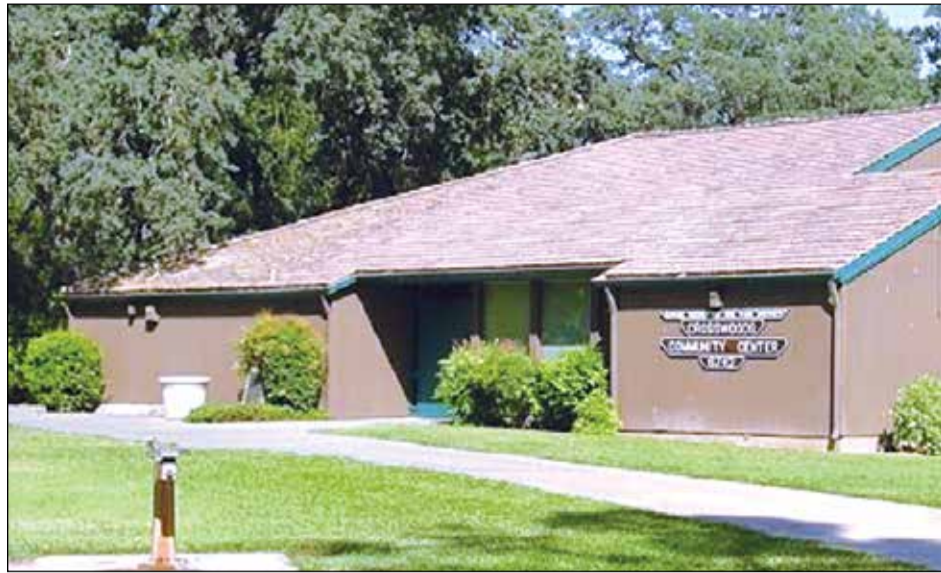
The Crossroads Community Center behind the Sylvan Library at 6742 Auburn Boulevard is the preferred location for a planned Meals on Wheels senior cafe. Photo courtesy of Sunrise Recreation and Parks District
