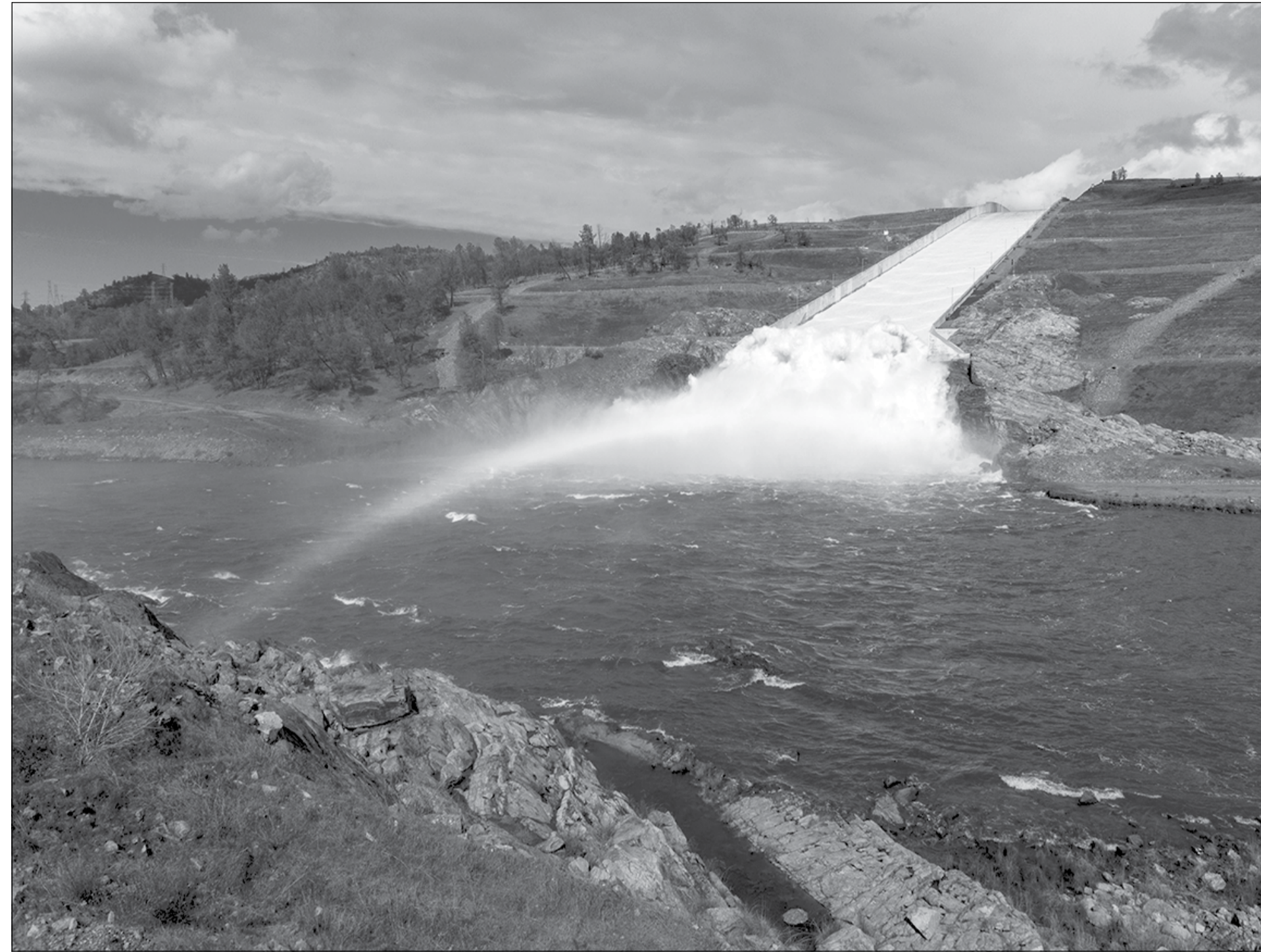
Storms have arrived in California. The Oroville Spillway at Lake Oroville in Butte County is ready for a wet year. Photo courtesy California Department of Water Resources
