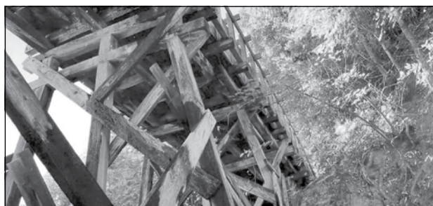
The Hell 4 Stout Flume helps maintain water deliveries for the purpose of irrigation in North Yuba Water District. Photo courtesy of Yuba Water Agency
