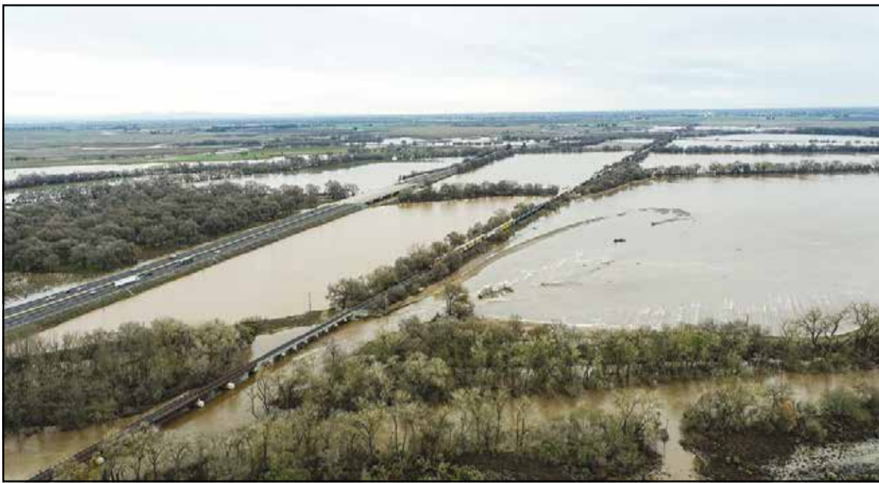
A drone photograph of the flooded lands along Highway 99, north of Galt, on Jan. 2. That portion of the highway was reopened after floodwaters receded from it. Photo by Tim O'Hara
