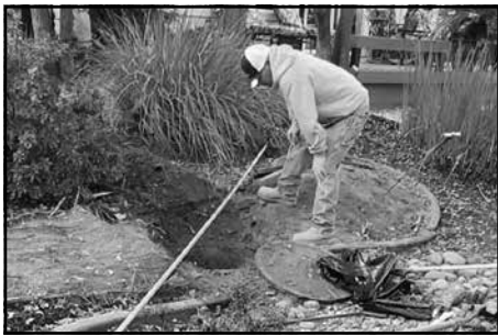
Image shows the open manhole, the cover, and some of the matted roots found inside.
