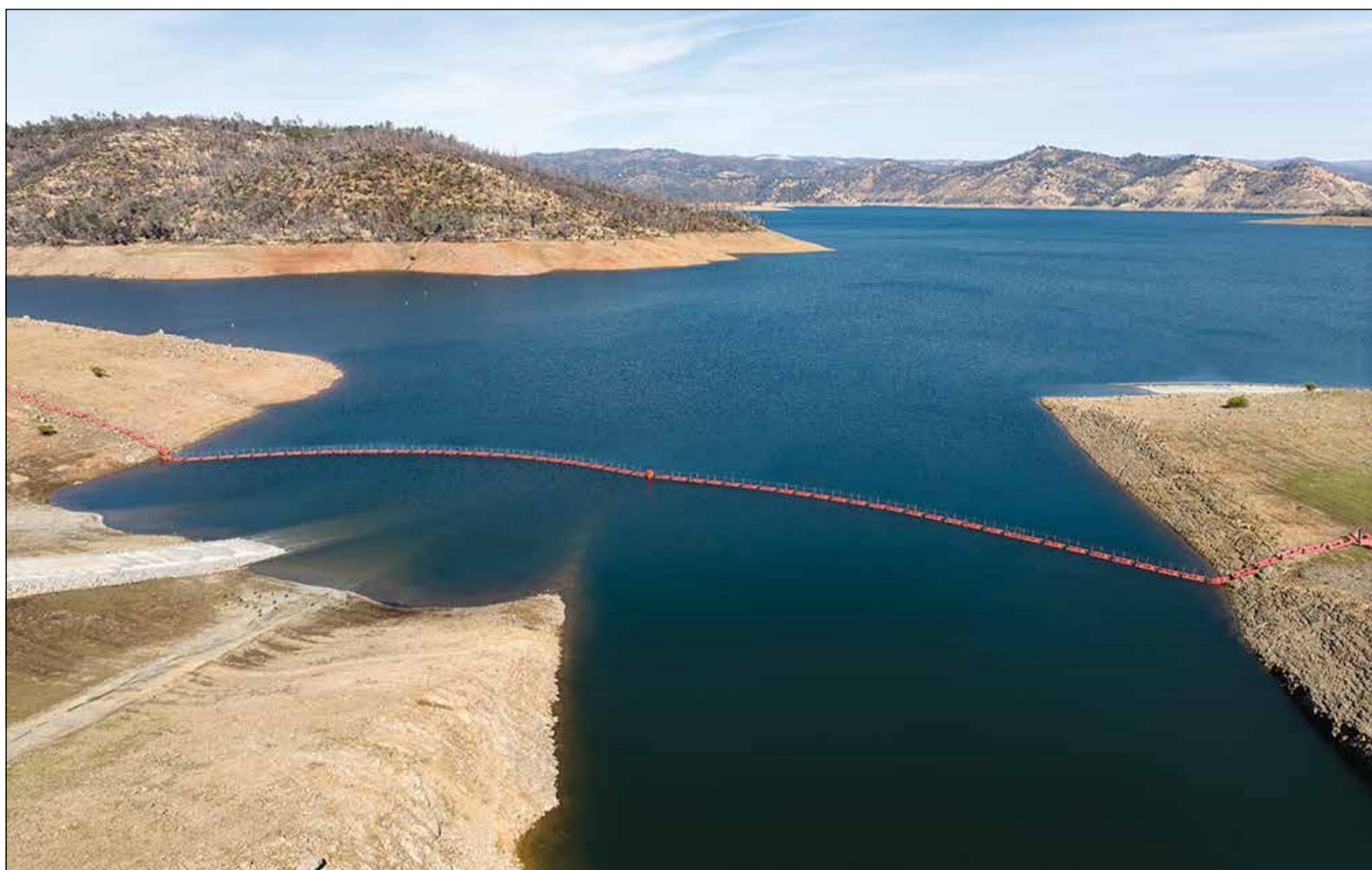
A drone view of water levels at the Oroville Dam located at Lake Oroville in Butte County, California. On this date, the water storage was 2,581,728 acre-feet (AF), 73 percent of the total capacity. Photo taken October 2, 2023. Photo by Fred Greaves/California Department of Water Resources
