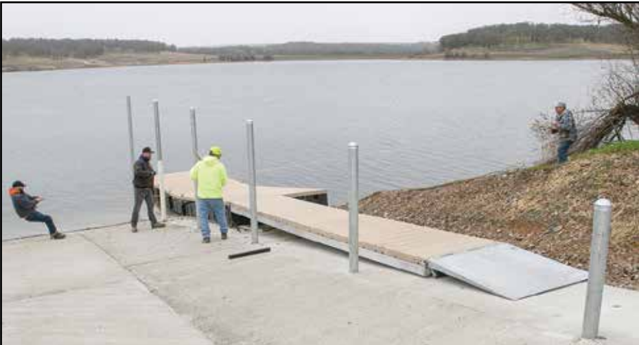
Rancho Murieta Association Maintenance Department employees launch a new boat dock at Lake Calero on Jan. 9. The RMA employees built the new concrete ramp first. Photos by Gail Bullen
