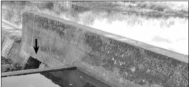
The photo shows a hole in Granlees Dam at the top of the fish ladder that had been blocked by a chair and a hefty branch. The National Oceanic Atmospheric Administration asked CSD to clear the blockage so fish could get through.
