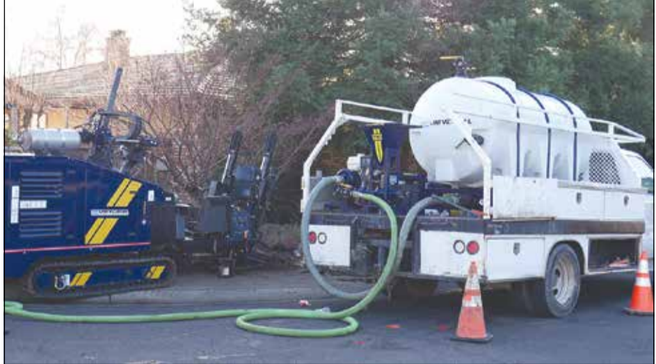
Equipment used to place fiber optic lines is shown here.
