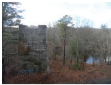
Triad bridge abutment
