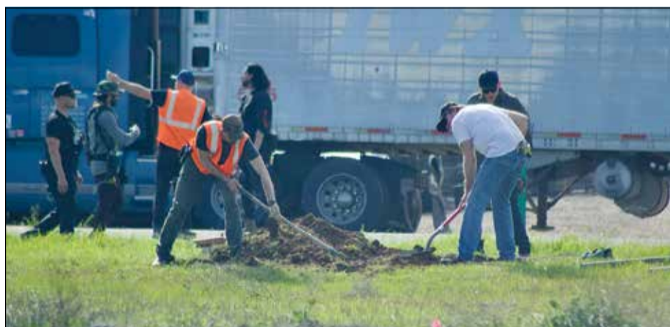
Film crews dig space near the Union Pacific railroad tracks to lay a camera dolly track.
