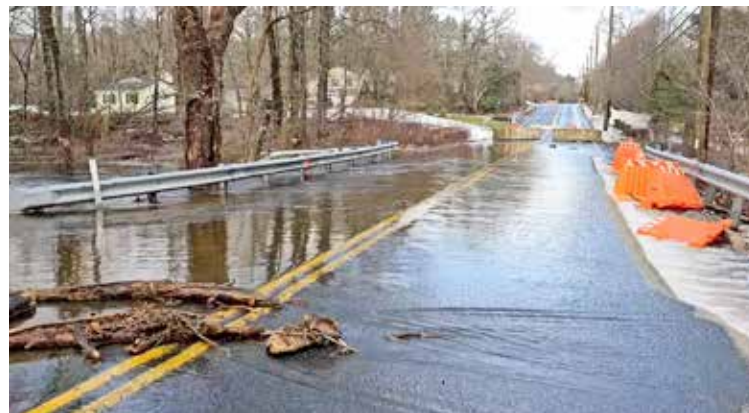
Flooding, like that seen January 10 on Providence Street in Mendon, also damages basements. Photo courtesy of Nicholas Miller
