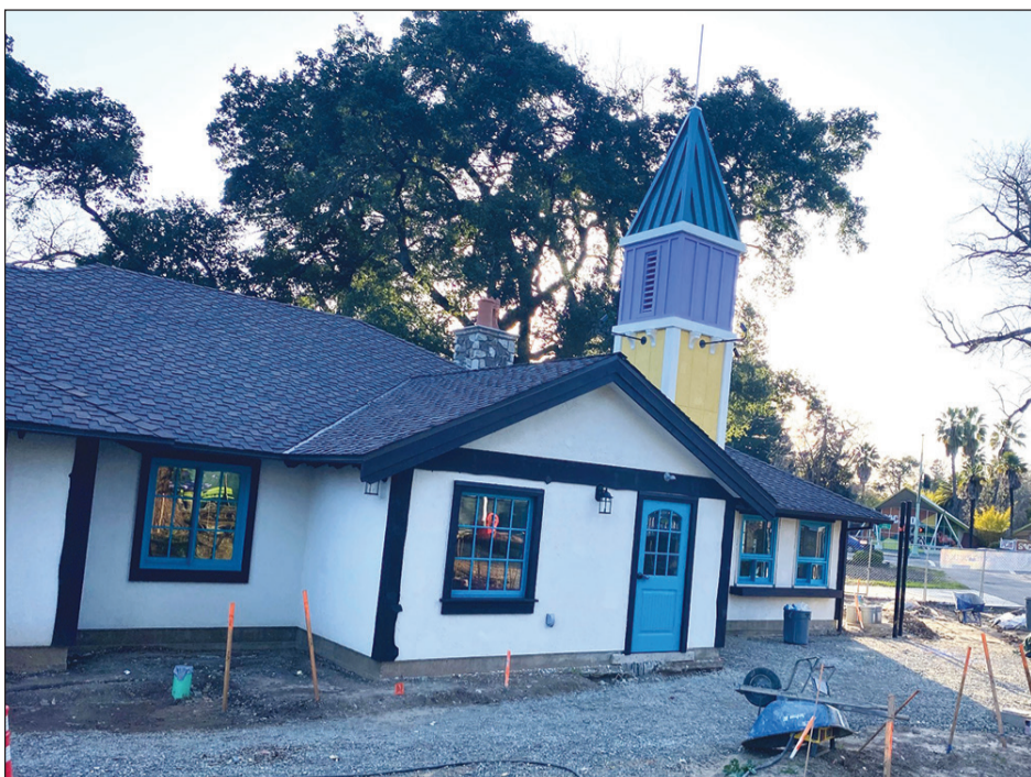
The new welcome center is almost complete.
