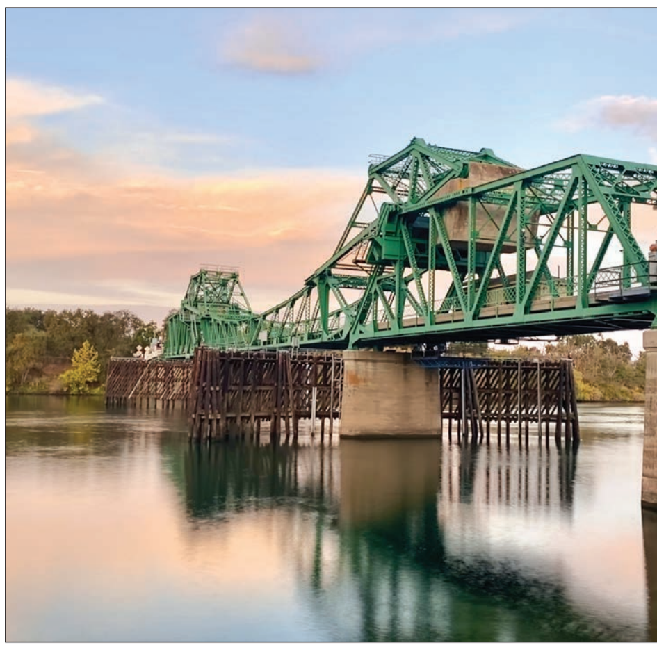
Bridge over peaceful water...Freeport Bridge in Clarksburg.
