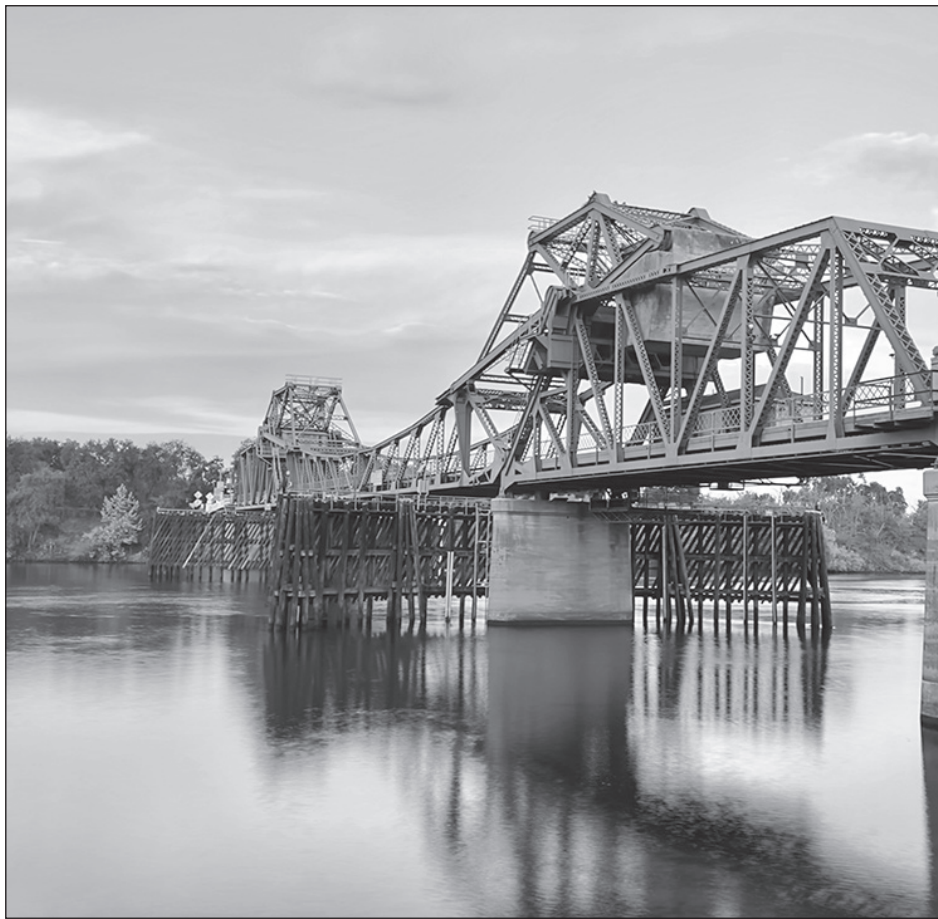
Bridge over peaceful water...Freeport Bridge in Clarksburg.
