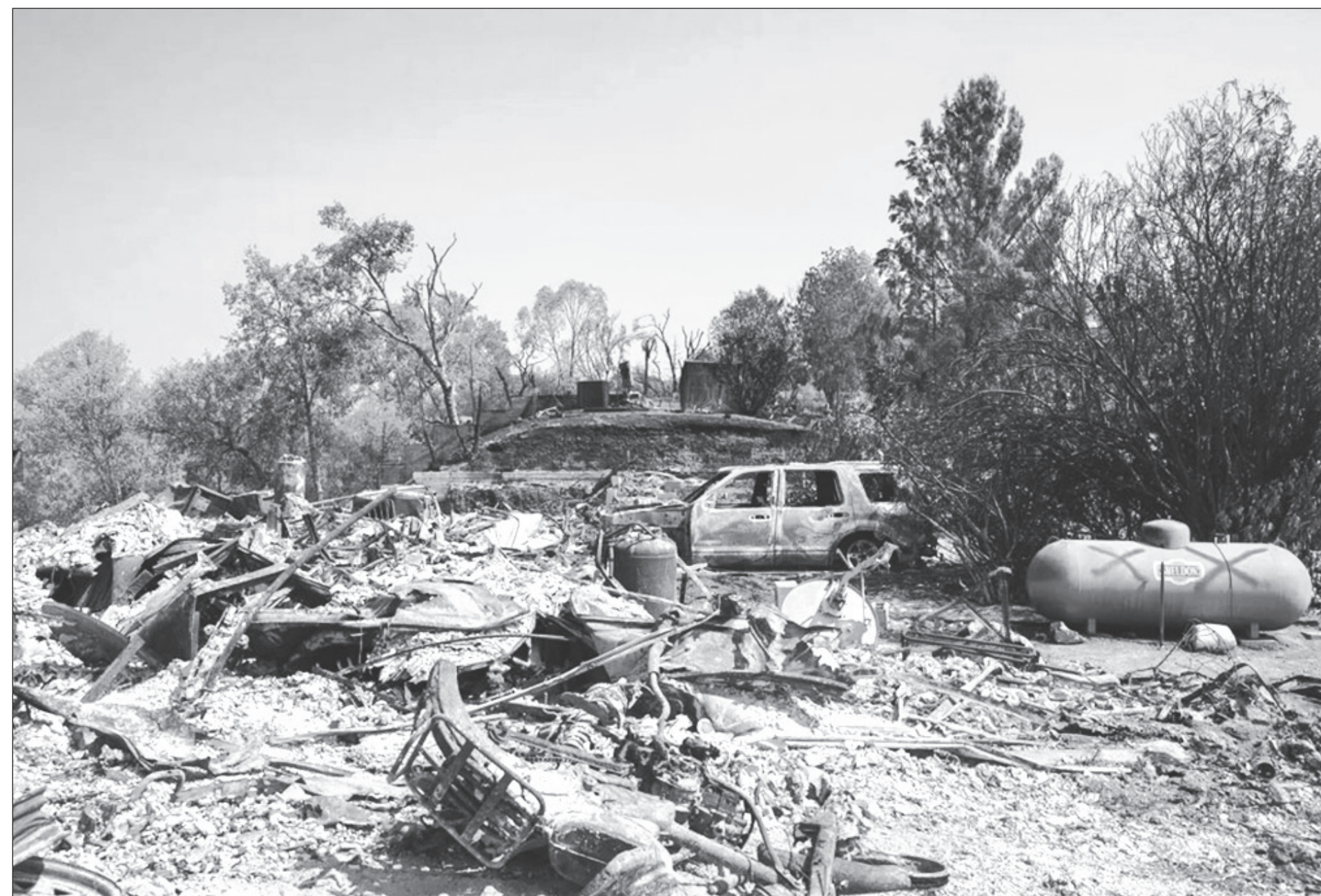
Here are the remains of a burned home in Berryessa Highlands on Sept. 21, 2020. Photo by Anne Wernikoff for CalMatters
