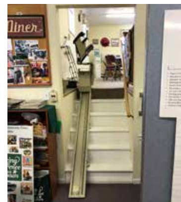
The second floor of the current Mendon Senior Center is accessible by this single stairway and stair lift. Photo credit: Theresa Knapp
