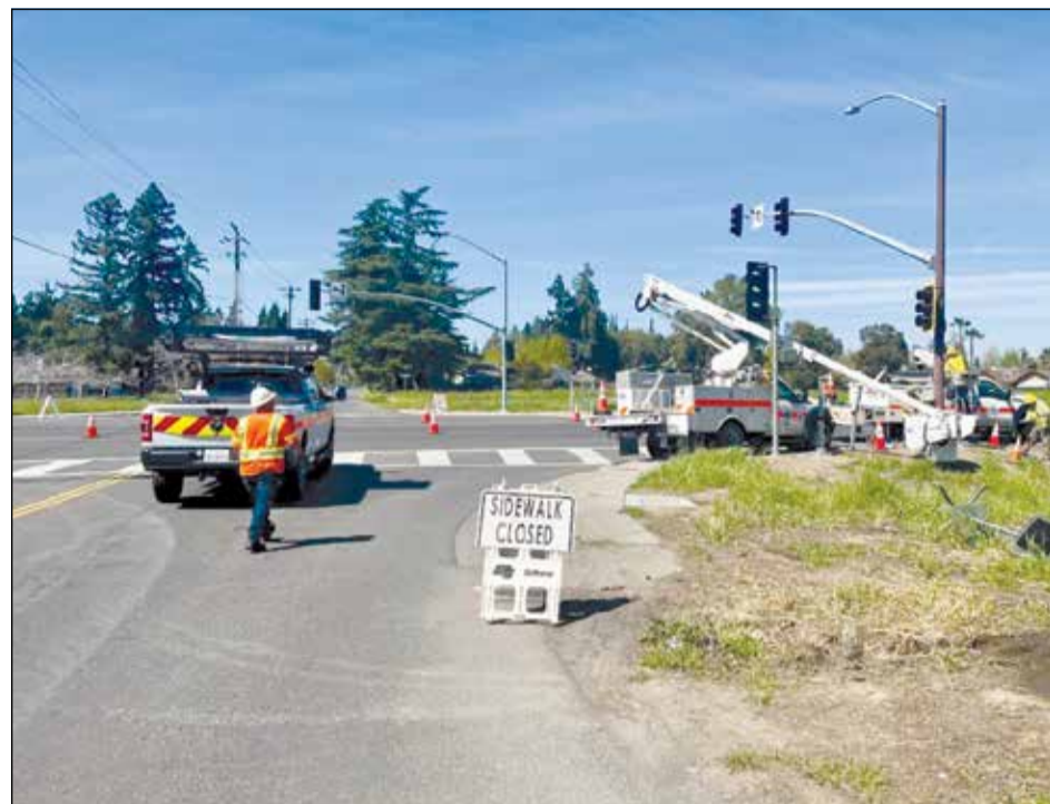
Workers move fast to make the repair. Photo courtesy of Caltrans
