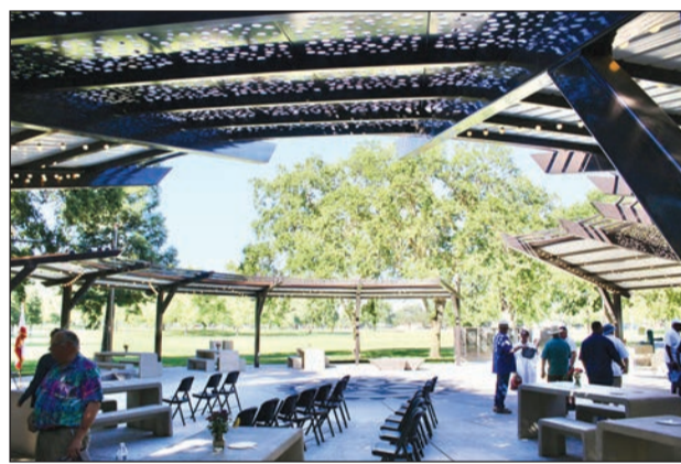
The refurbished Rotary Grove features steel shade structures designed to give “dappled shade” and a concrete picnic area.
