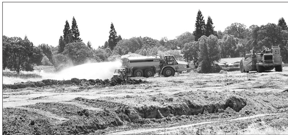
Although trucks providing dust control at the Residences East and West subdivision use potable water, the effects on the water tanks are minimal. Photos by Gail Bullen
