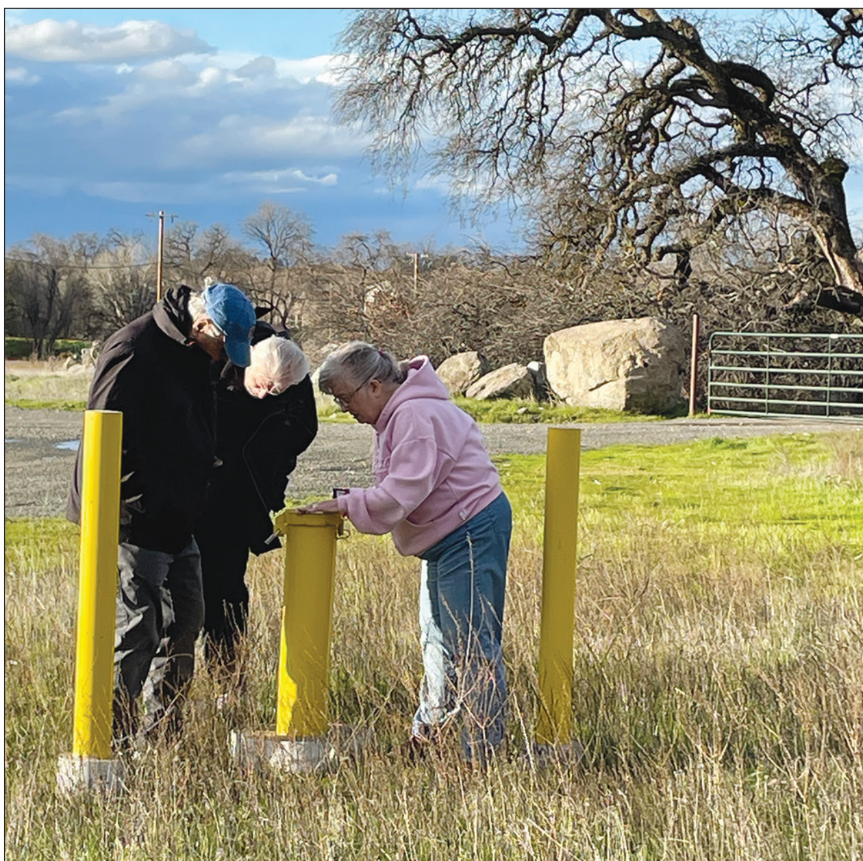
From left, Lincoln City Councilman Bill Lauritsen, Ray Birge and Anne Constantin Birge, members of the grassroots Titan 1-A Missile Site Environmental Contamination and Remediation Committee, were looking at the number of the monitoring well to see what the trichloroethylene (TCE) levels have been over the years. Photo by Carol Feineman
