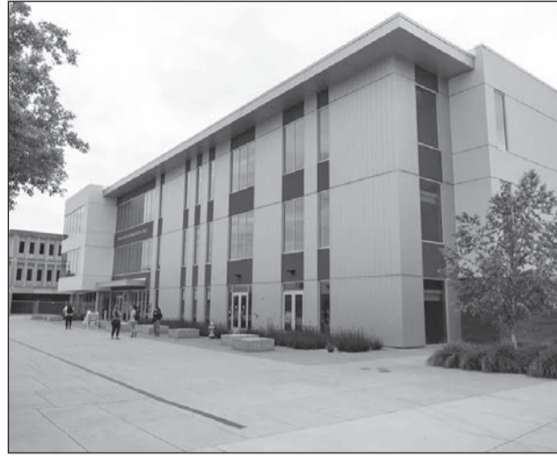
The Diane Bryant STEM Innovation Center at American River College. Cosumnes River College also has a MESA program. Details at crc.losrios.edu/student-resources/mesa .
