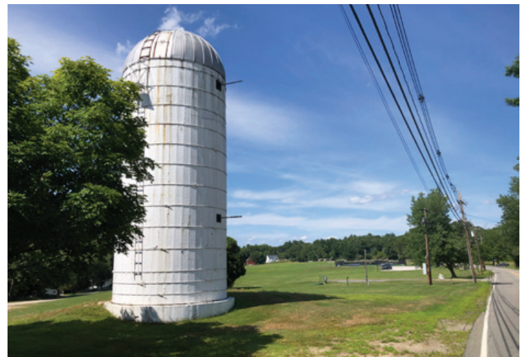
The site of the former Henry Warren Milking Barn which will be reconstructed in its original location to benefit the town and Framingham State University. Photo credit: Theresa Knapp
