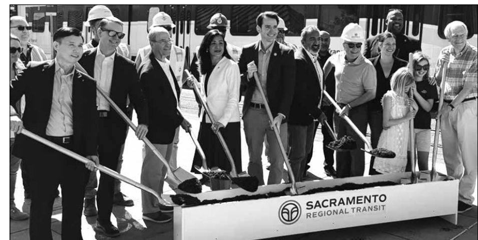
Assemblyman Josh Hoover, his team, and Sacramento Regional Transit District are at the Watt/1-80 Transit Center Improvement Project. Courtesy photo of Assemblyman Josh Hoover
