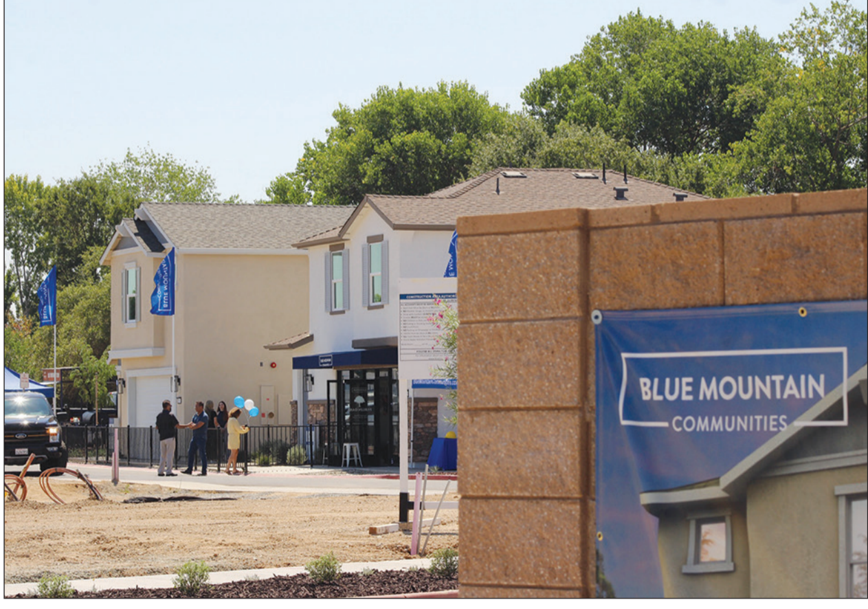
The Parlin Oaks housing development on Walnut Avenue and Carillion Boulevard held a grand opening event, showing its two model homes. Photo by Matthew Malone
