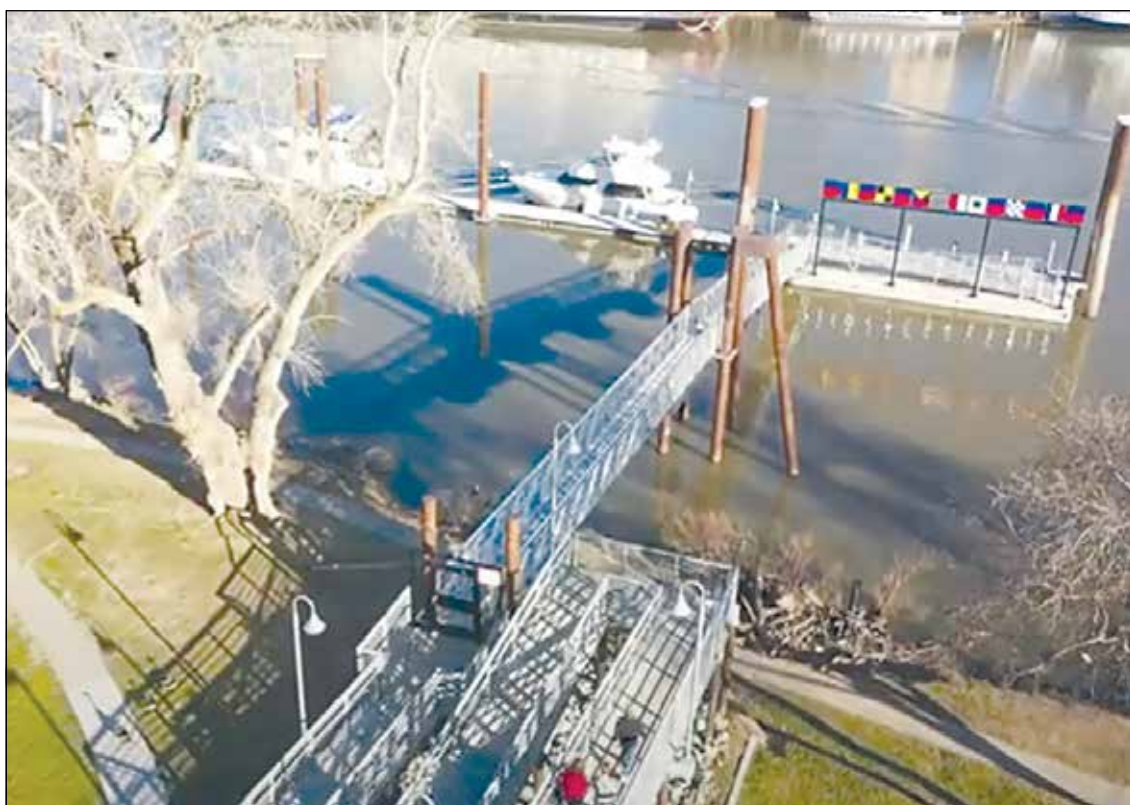
Here is an aerial view of the Etenesh Zeleke Public Dock on the Sacramento River, dedicated to an Ethiopian immigrant and long-time resident. Photo courtesy of the City of West Sacramento
