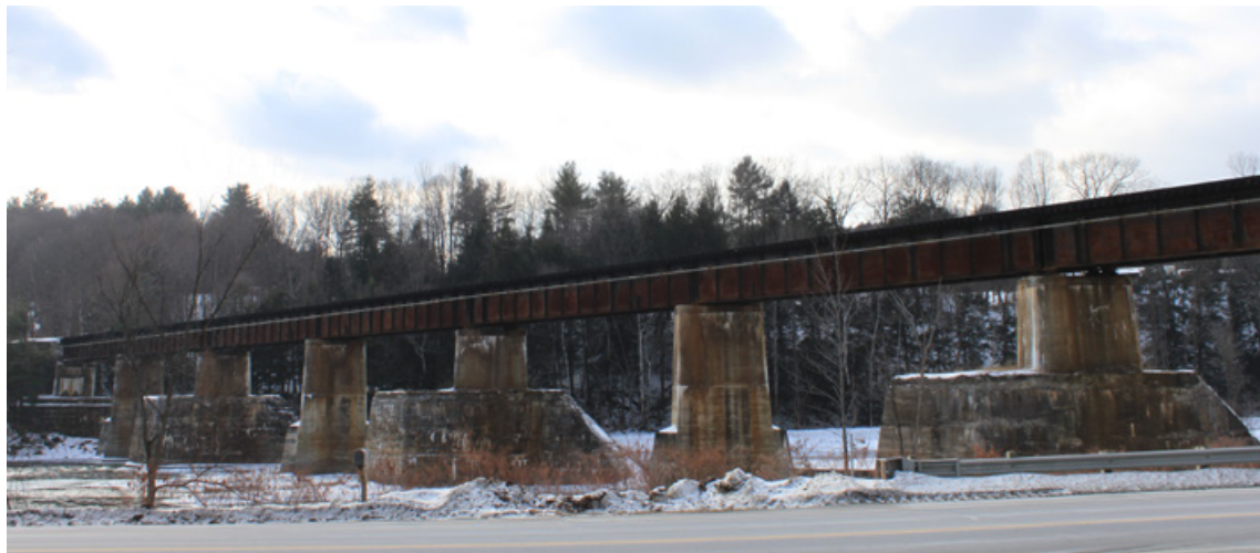
Hartford Railroad Bridge. Photo courtesy of Bob and Vickie Hughes
