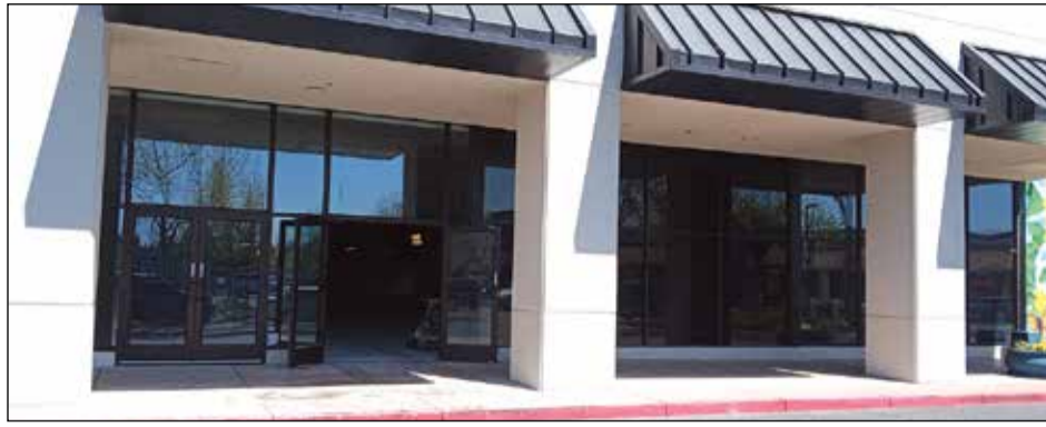
The new 25,020 square-foot HomeGoods store in Citrus Heights fills a space labeled "6130A" which was previously occupied by Stein Mart.
