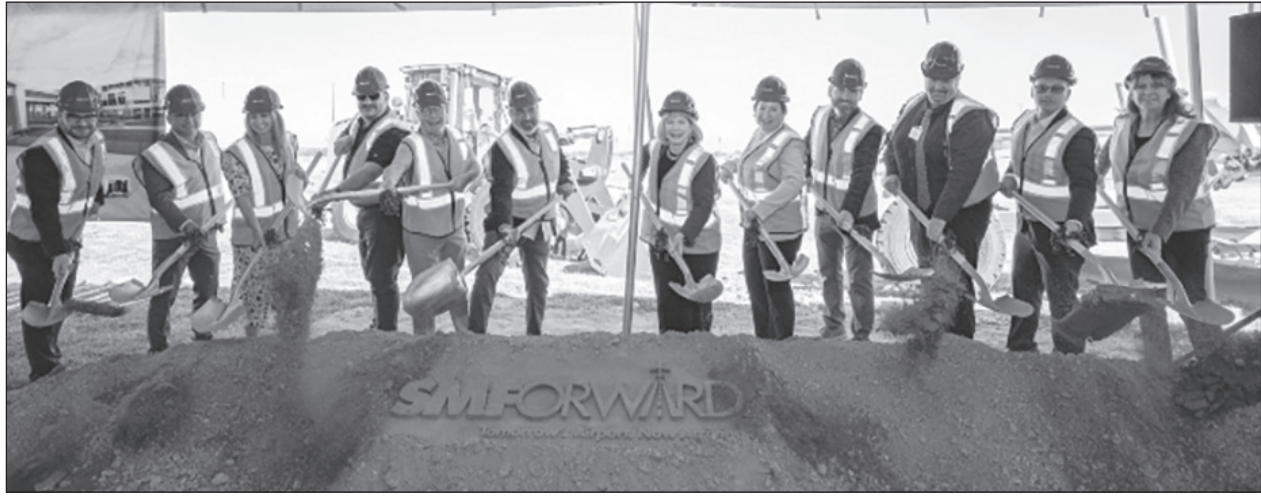
The new walkway will connect Terminal B to Concourse B. Photo courtesy of Sacramento County
