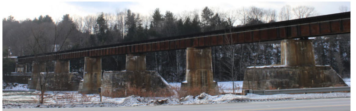
Hartford Railroad Bridge. Photo courtesy of Bob and Vickie Hughes
