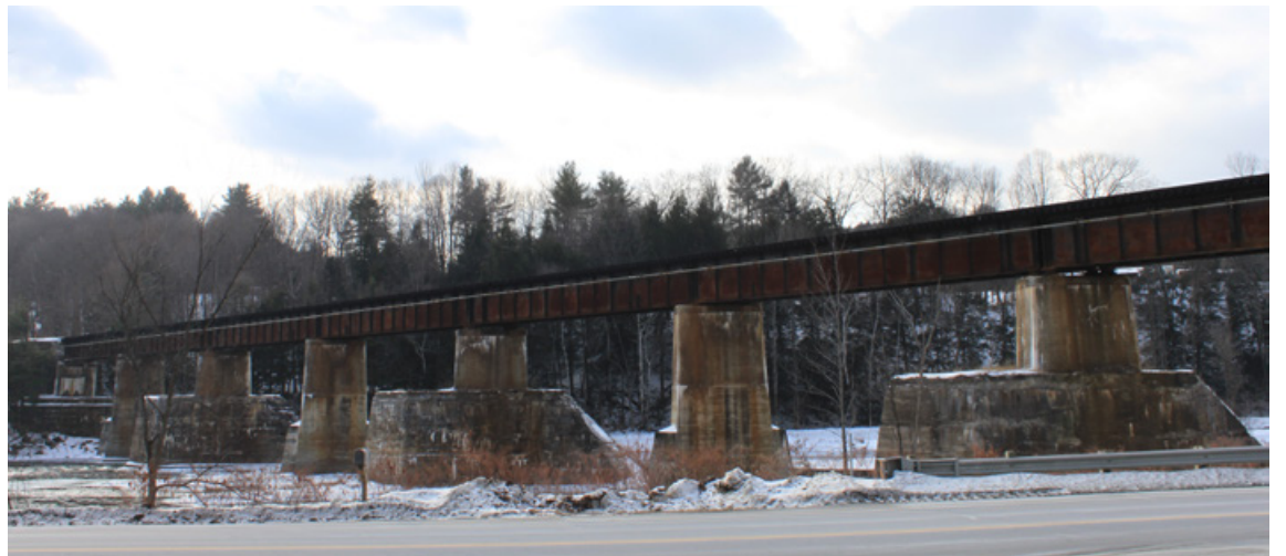
Hartford Railroad Bridge. Photo courtesy of Bob and Vickie Hughes
