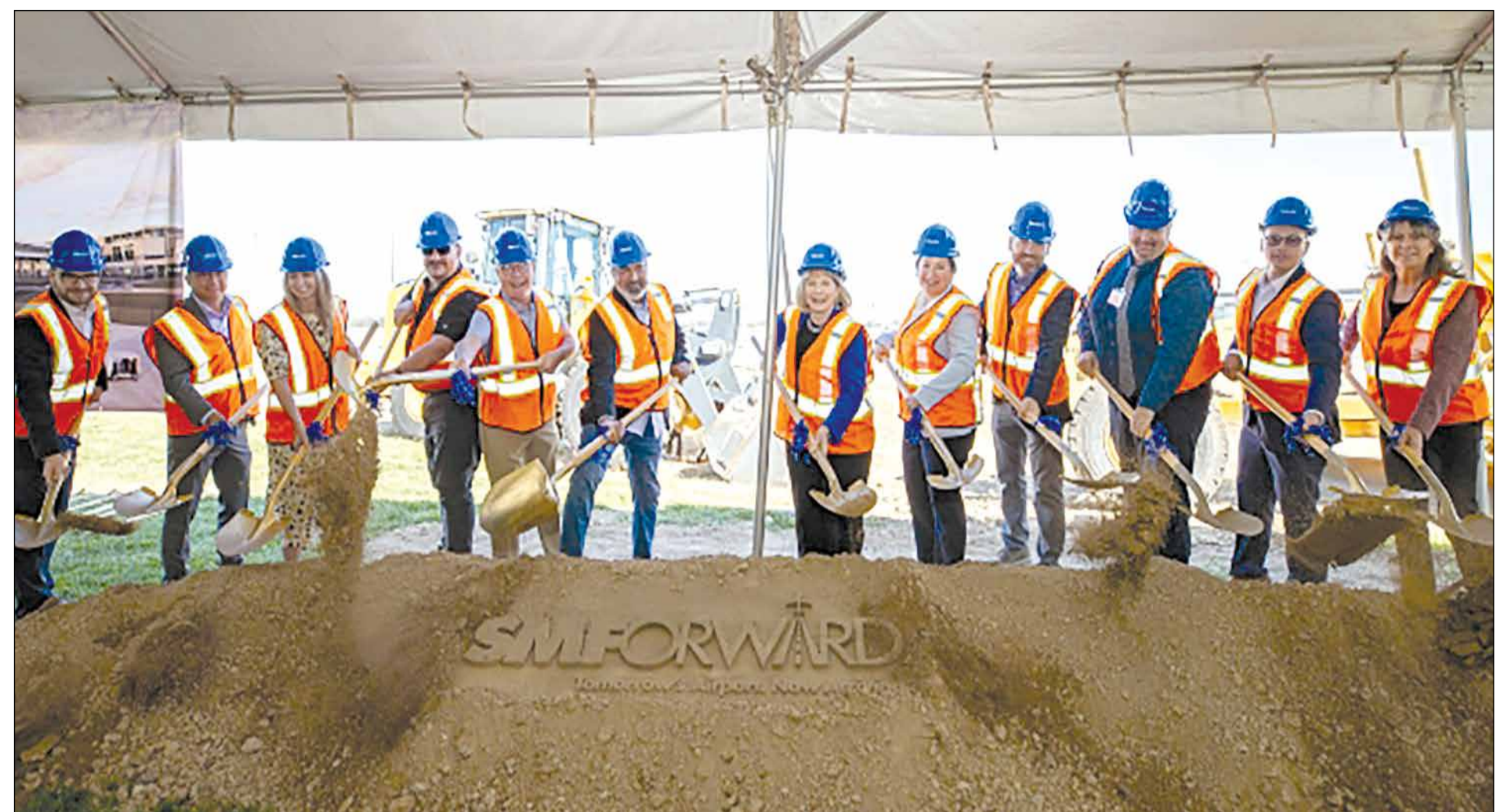
The new walkway will connect Terminal B to Concourse B. Photo courtesy of Sacramento County
