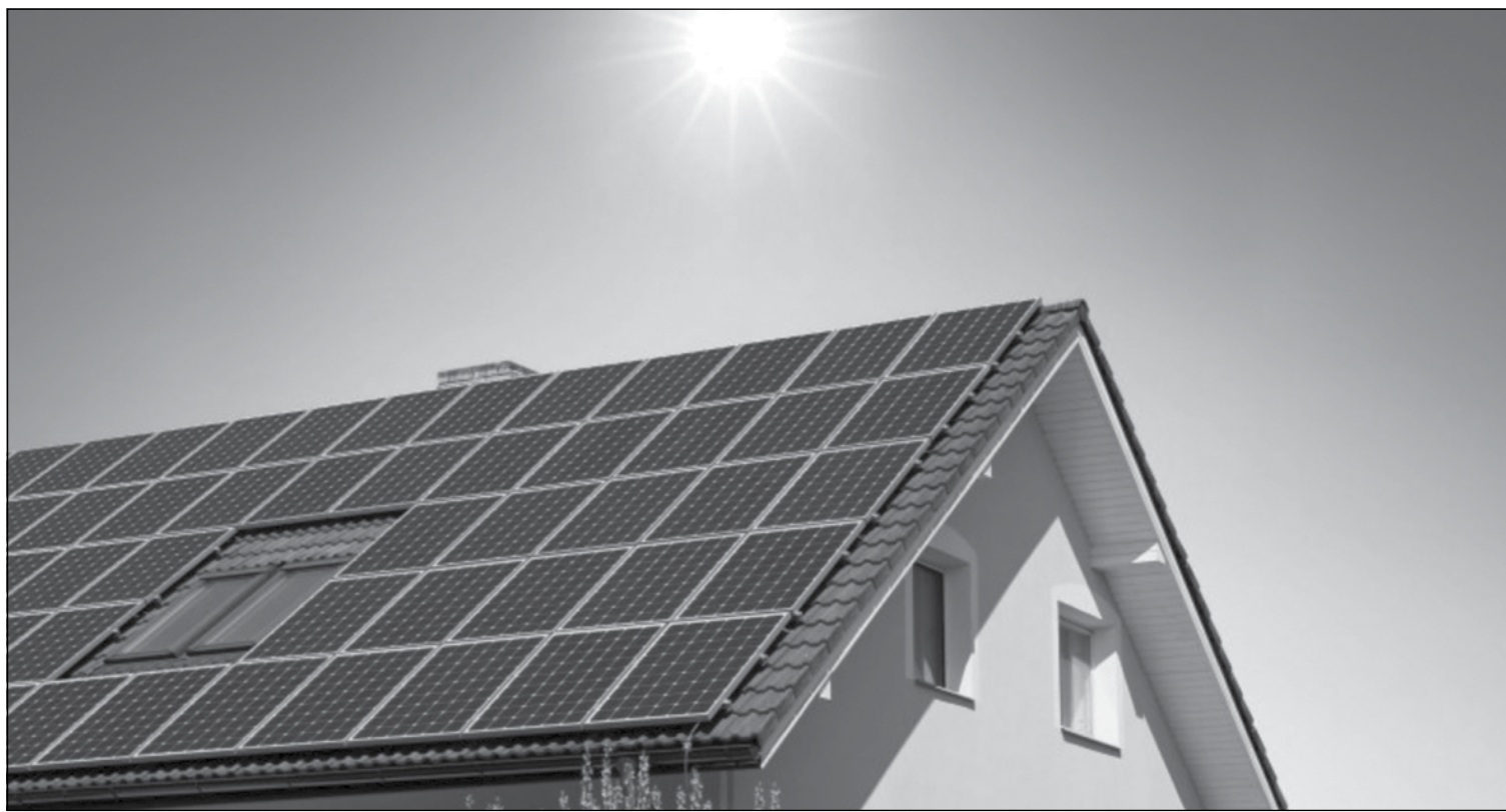
Rooftop solar. Photo provided by www.energy.gov
