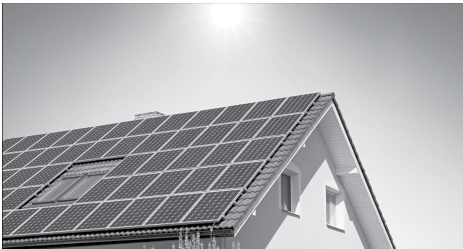
Rooftop solar. Photo provided by www.energy.gov
