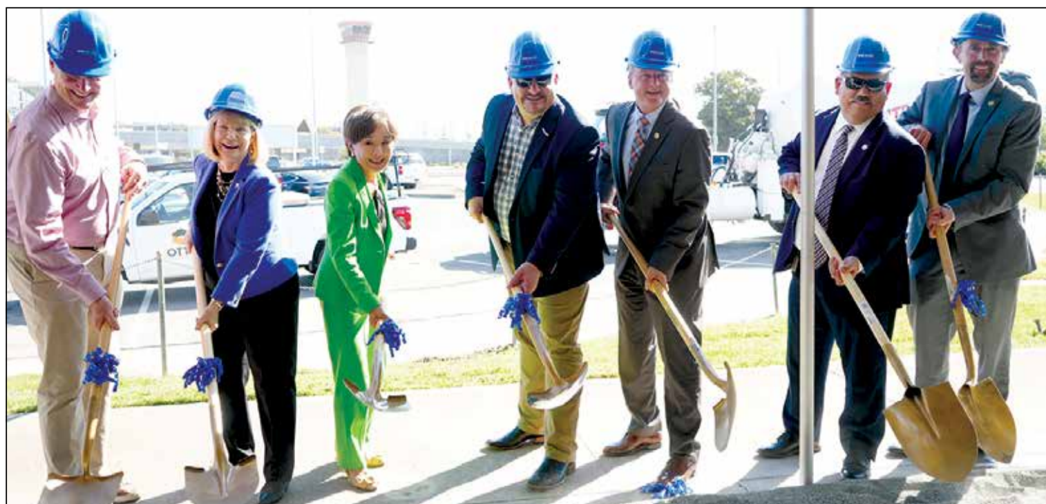
Airport officials, along with local dignitaries, break ground for the new Terminal B parking garage. Photo courtesy of Sacramento County Department of Airports
