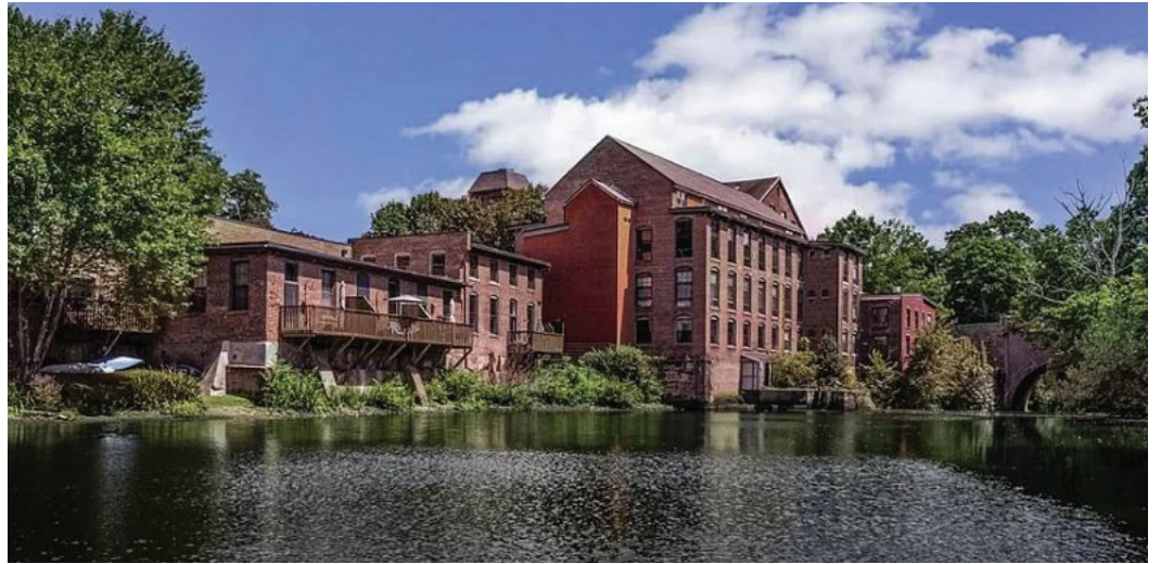
The 1-bed, 1-bath, 686-square-foot unit at 14 Sanford Street, Unit 46, in Medway recently sold for $270,000. Image credit: www.zillow.com
