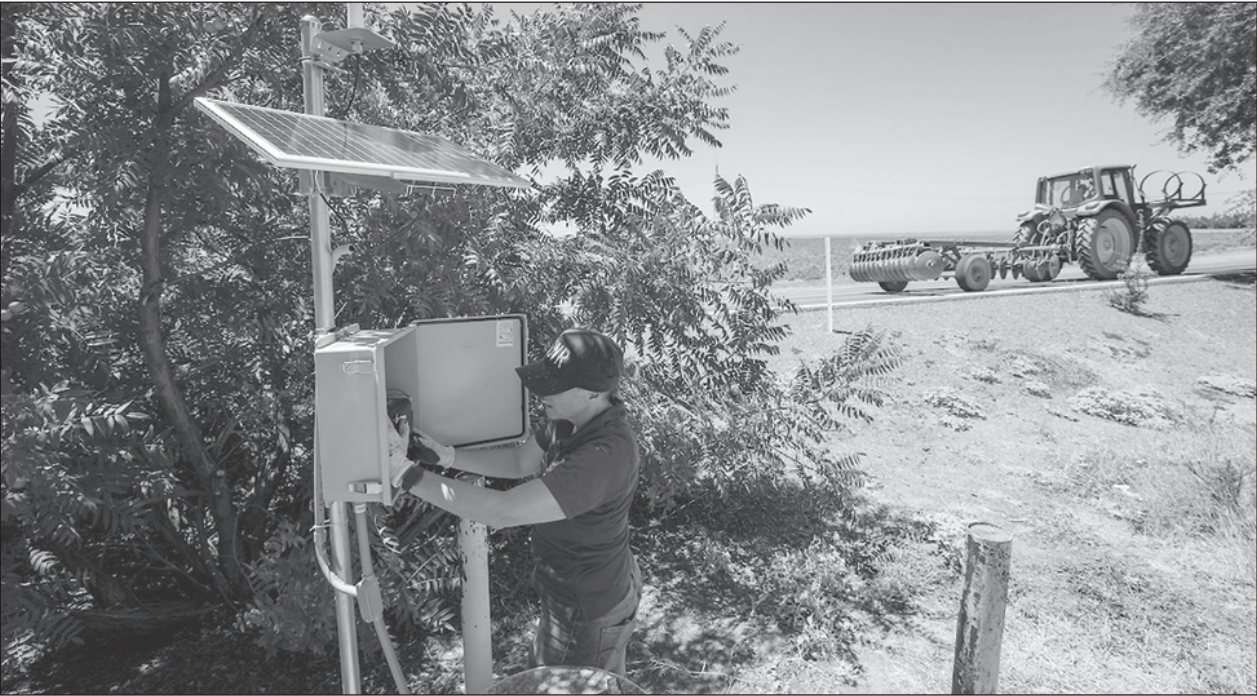
California Department of Water Resources employee Katy Janes, Groundwater hydrogeologist in the Geology and Groundwater Investigations Section of the Division of Regional Assistance North Central Region Office, installs new telemetry equipment in groundwater monitoring wells in Colusa County on July 24. Photo courtesy of California Department of Water Resources
