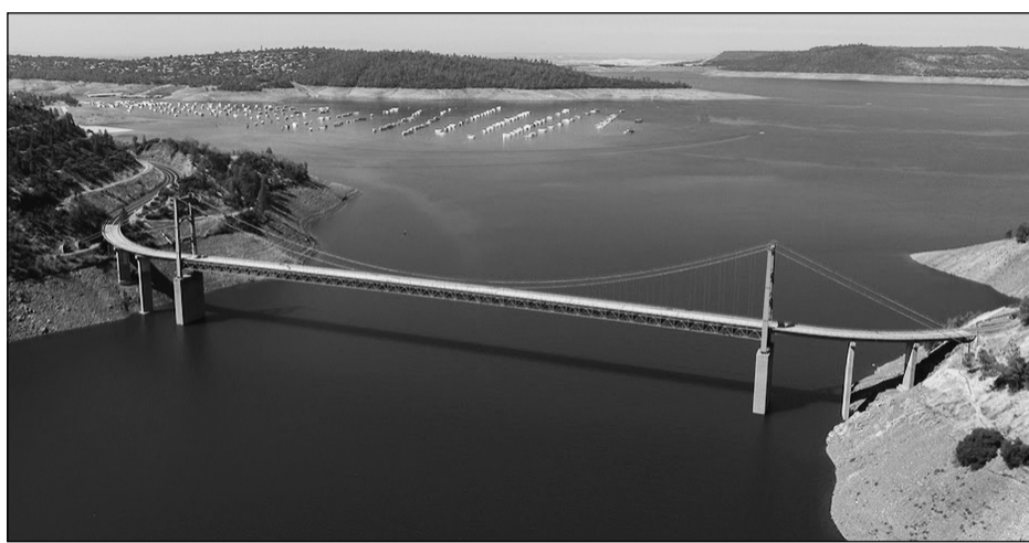
Pictured here is a drone photo of Lake Oroville taken Sept. 5. Photo courtesy of the California Department of Water Resources
