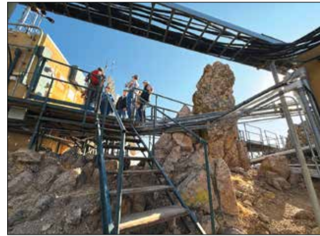
A series of staircases, catwalks and overlook decks lead to various access points to communication towers and equipment located on the peak of South Butte in Sutter County.
