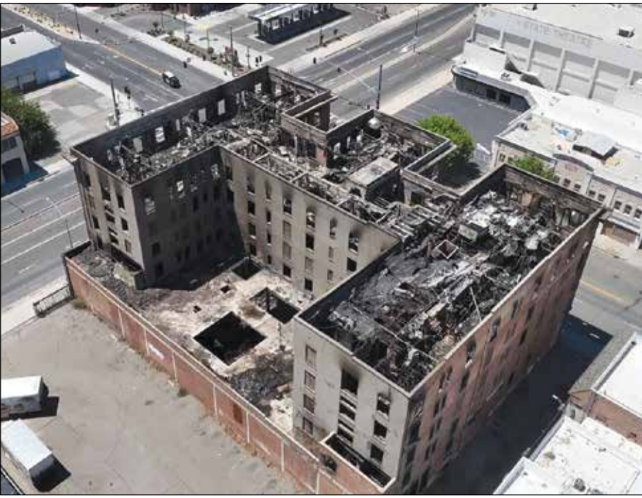
Nearly 6 months after fire destroyed the Hotel Marysville, demolition of its ruins began Wednesday, Dec. 11. Photo courtesy of the City of Marysville
