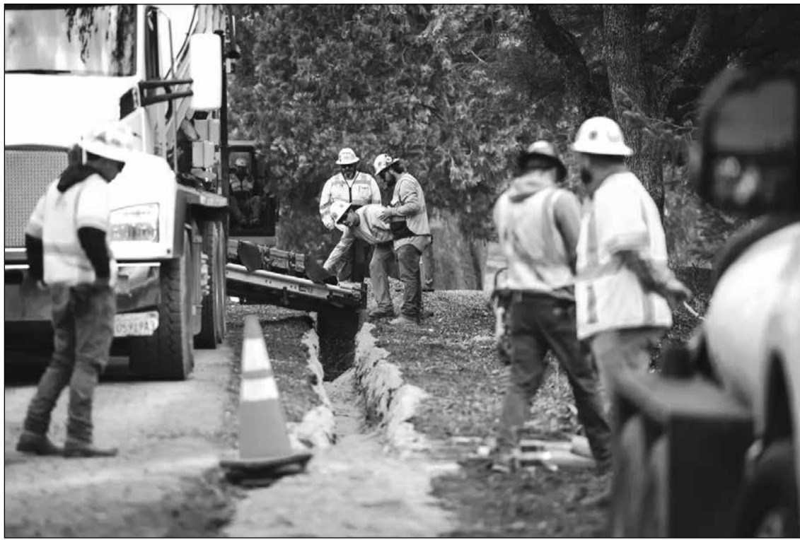
Contractors with PG&E work in a trench to lay underground electric cables in Placer County on Oct. 17. Burying lines and other wildfire prevention projects have raised the price of electricity in California. Photo by Miguel Gutierrez Jr., CalMatters
