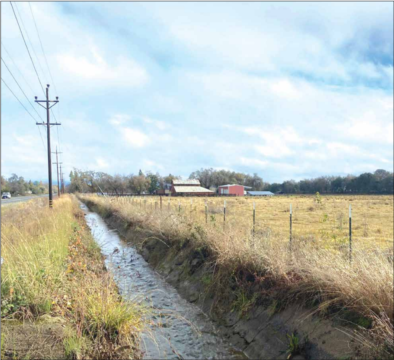
Pictured is a canal within the Hallwood Irrigation Company’s service area to be lined to reduce seepage and water loss. Photo courtesy of Hallwood Irrigation Company
